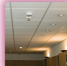
Acoustic ceiling tile
